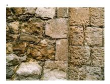
The picture on the left illustrates two forms of ragstone galleting in one building, being part random stonework of the late 18th century and part later squared and coursed work. In the centre are quoin blocks that are block bonded into the random stonework to form a corner. Galleted Kentish ragstone masonry can be found in a narrow band from Deal in the east, crossing Kent to Maidstone and Sevenoaks and heading west to Surrey.
